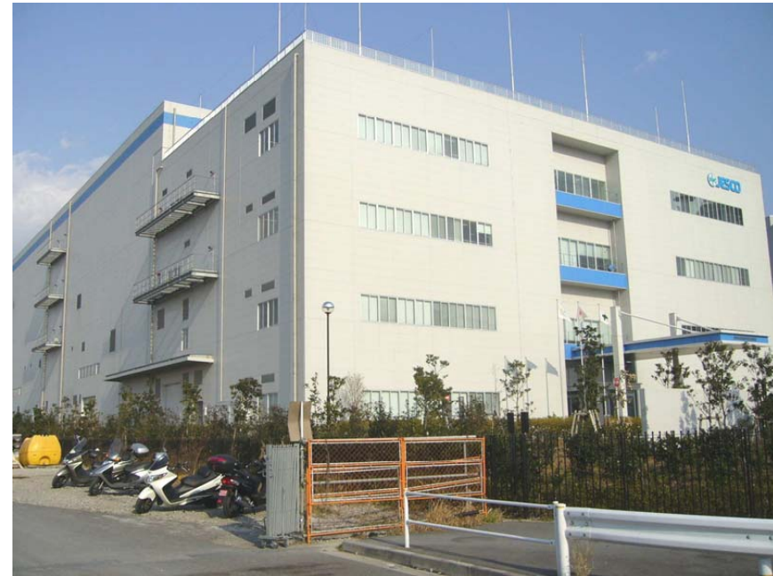
JESCO's Tokyo Facility for PCB Waste Treatment
